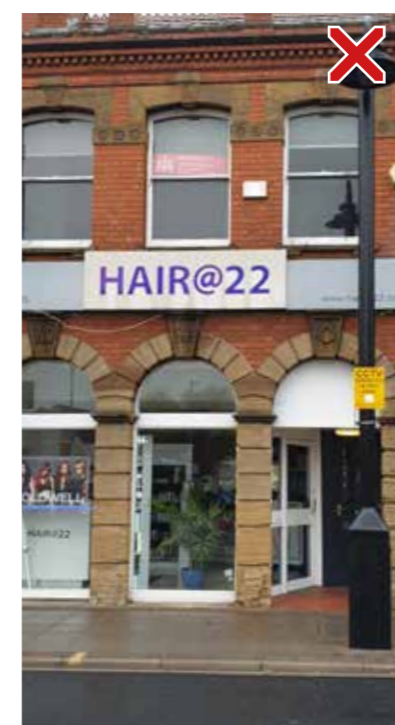
Projecting sign that overshails details on the original window
