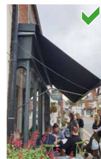
Blind box installed above cornice and fascia
