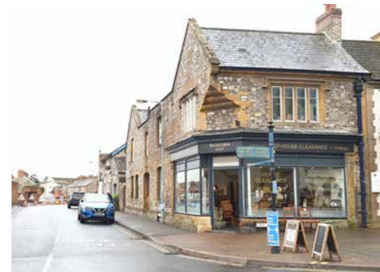
Boden Street Corner - present day
