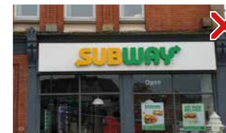
Oversized Fascia sign with overly large lettering detracts from the uniformity of the streetscene.
