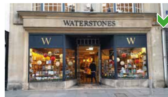
Individual mounted letters set on fascia working within existing dimensions. Opaque transom light, used for signage.
