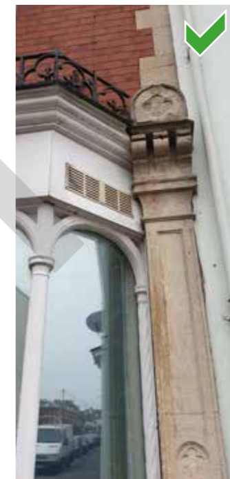
stone pilaster, ornate corbel and capitol at head all remains in-situ
