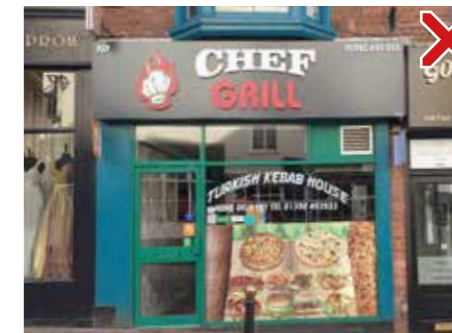
Signboard applied disregarding the detail of the window cill above
