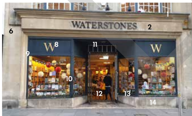
Left: Late 20 th century interpretation of the shop front Employing original intent, pilasters insinuated with a string detail, incorporating the cornice and fascia in stone within the elevation.
