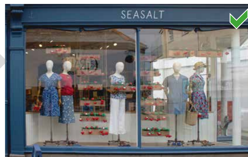
Large plate glass, set within original shop front, vertical separation maintained to introduce scale
