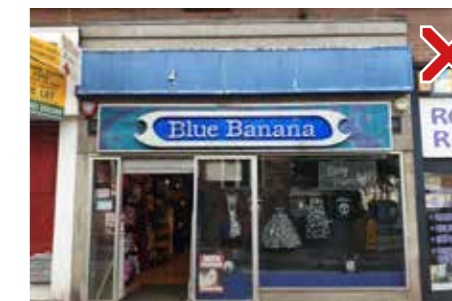
Two fascias applied obscuring the original design and intended position of the signage, lower set over original blind box
