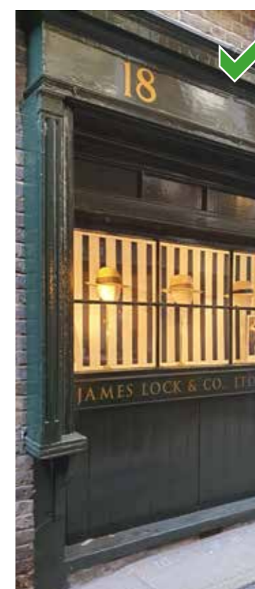
timber pilaster supporting fascia, with no capitol.
