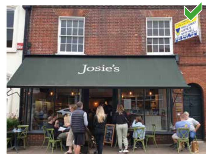
Example of blind advertising the shop front, working in tandem with the building design
